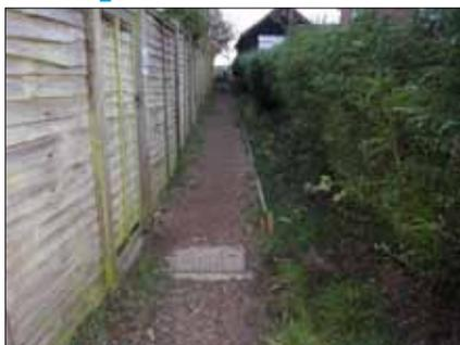
With materials from the Parish Council and with help from the Community Payback Team (supervised unpaid work by offenders), the section of footpath 1 next to The Old Forge in The Street has been repaired and a step up installed to make it easier to climb over the stile. The adjacent ditch was also restored to improve drainage.
